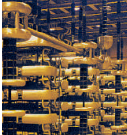
Page 25 Verifying HVDC thyristor design
