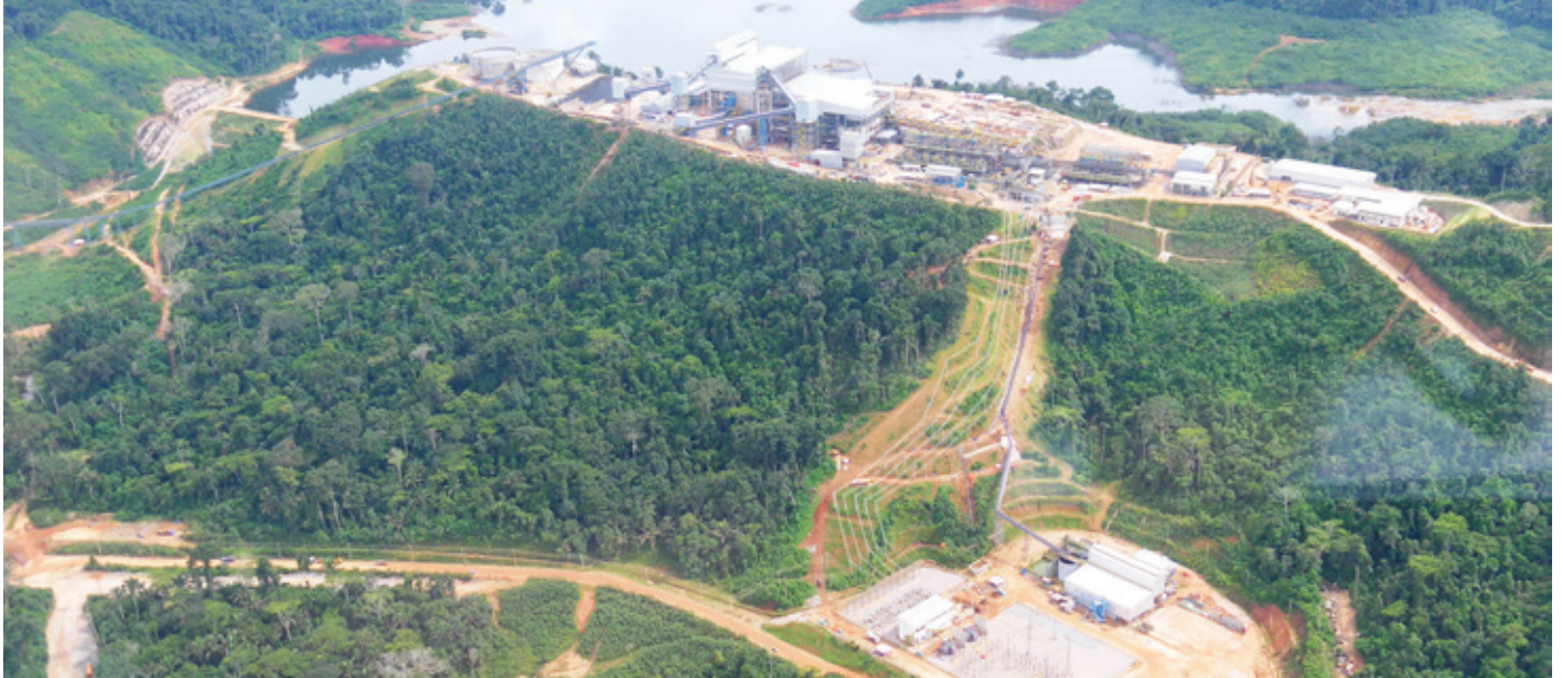
Vale's Solebo copper mine in Brazil, utilizing the System 800xA IEC 61850 solution.
