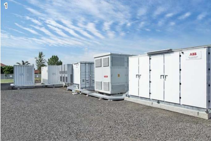
1 The GESS is installed in an industrial estate in northern Melbourne, Victoria, Australia, and provides support to a local end-of-line feeder
