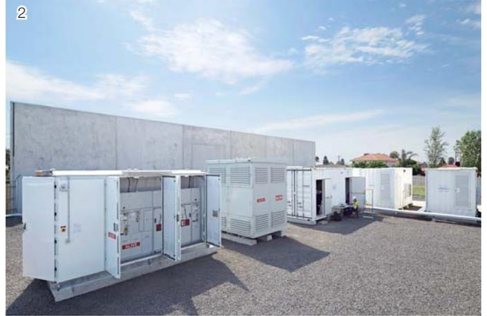
2 The GESS is fully portable, and all system components are transportable. The system is housed in six twenty-foot shipping containers and two transportable skids.
