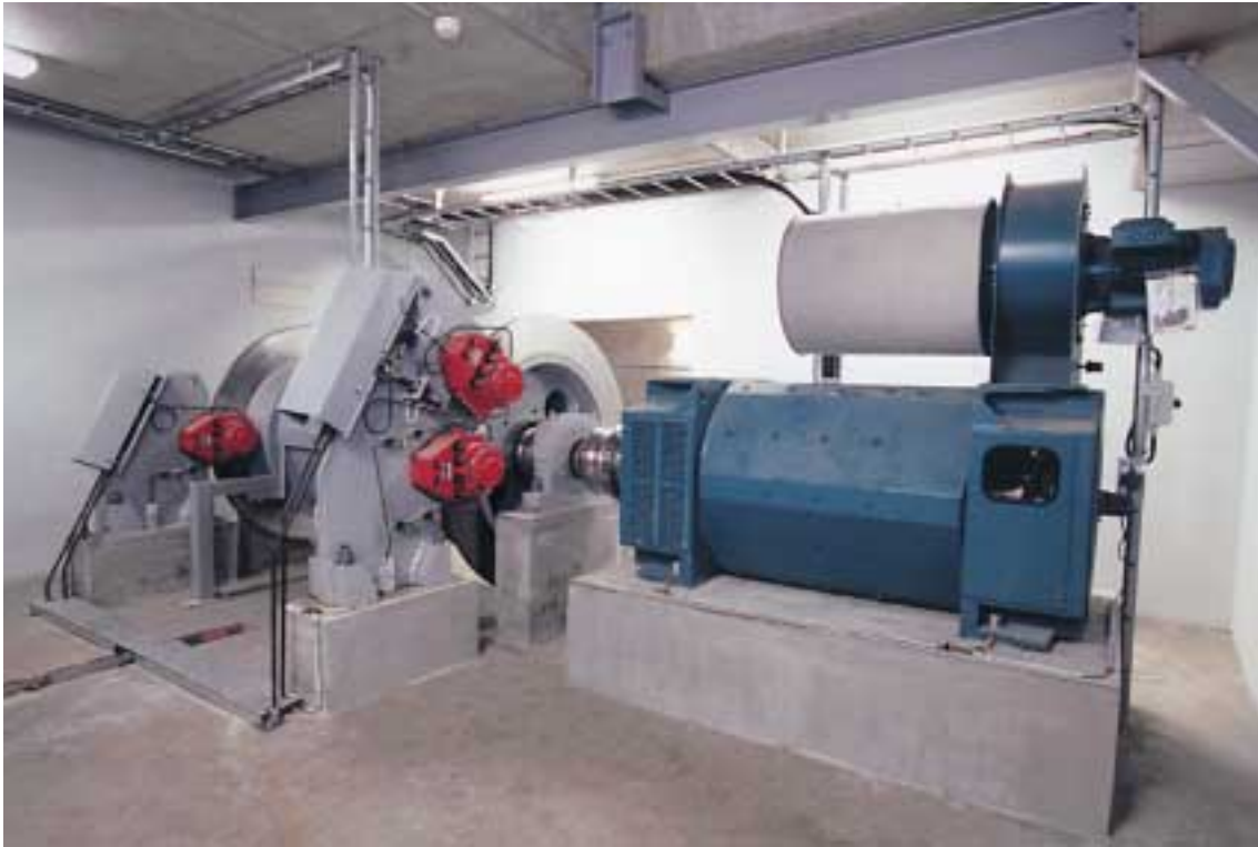
3 Each test track is equipped with two rope drives to facilitate control of the rope tension and bi-directional running of the track. The electric motors are controlled in terms of both speed and car position, and are able to deliver as much as 2x1750 kW of power during acceleration.
