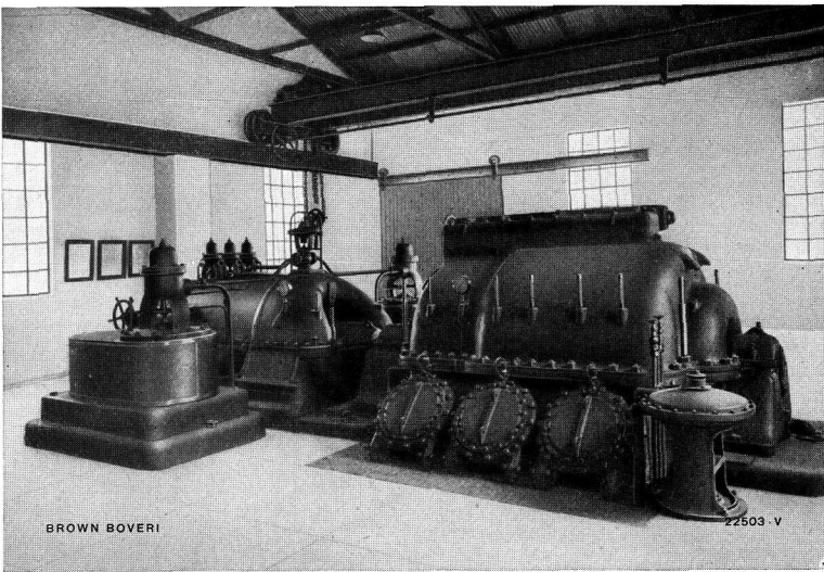
Fig. 3. — Single housing compressor having 3 intermediate coolers of V shape lodged in the lower part, 11 impellers, model 1915 (without water-jacket cooling). This design met with great success; it was a pioneering achievement which had many imitators.
