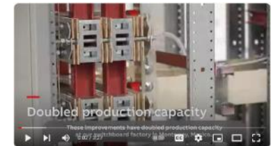
Efficiency & Innovation – Expansion of ABB switchboard operations
