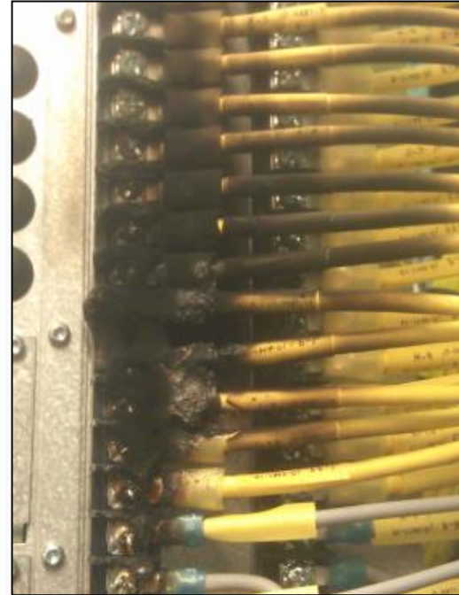
Damage due to CT arcing
