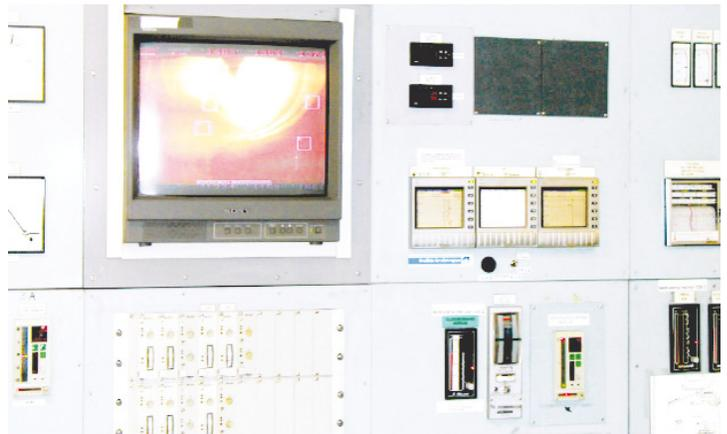
Figures 3-4 Wall panels with chart recorders, alarm enunciators and single-loop controllers.
