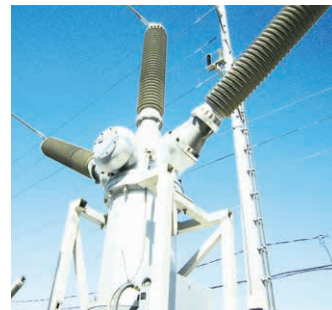
SF 6 -gas-to-air bushing to connect overhead lines
