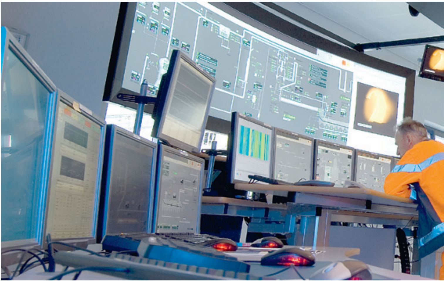
Control room at Jura Cement plant, located in Wildegg, Switzerland
