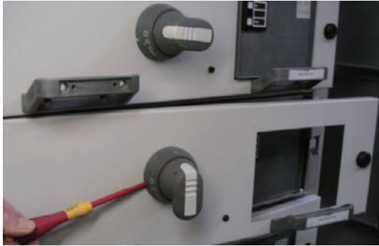
56 Unlatching the front cover of a withdrawable module by means of a screw driver
