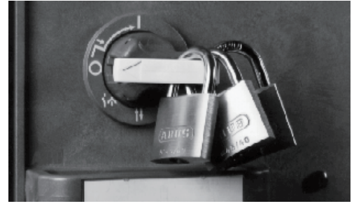
49 Withdrawable module size 8E/4 with 3 padlocks
