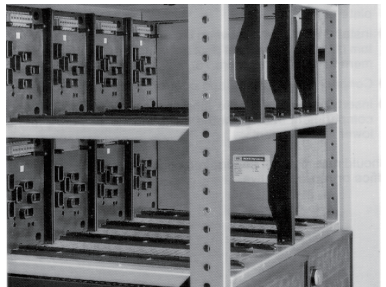
59 Conversion to withdrawable module compartments size 8E/4 and 8E/2
