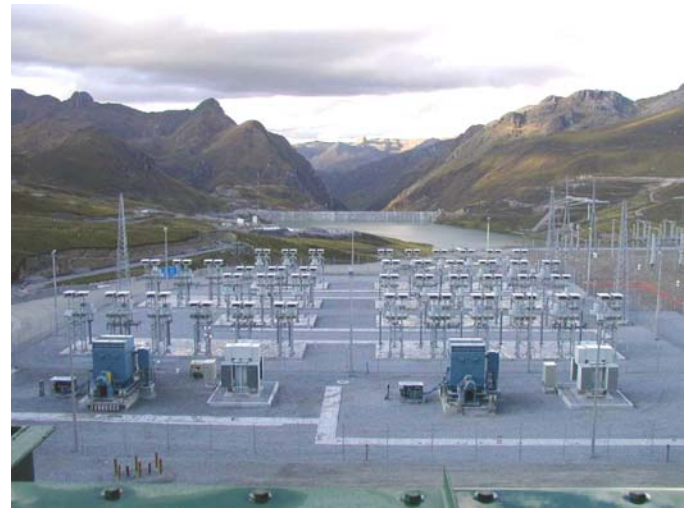
Figure 3. Filter installation at Antamina
