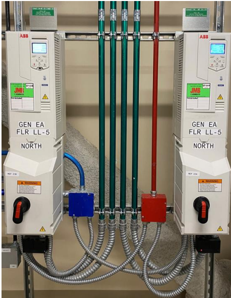
Figure 3: ACH580 with conduit
