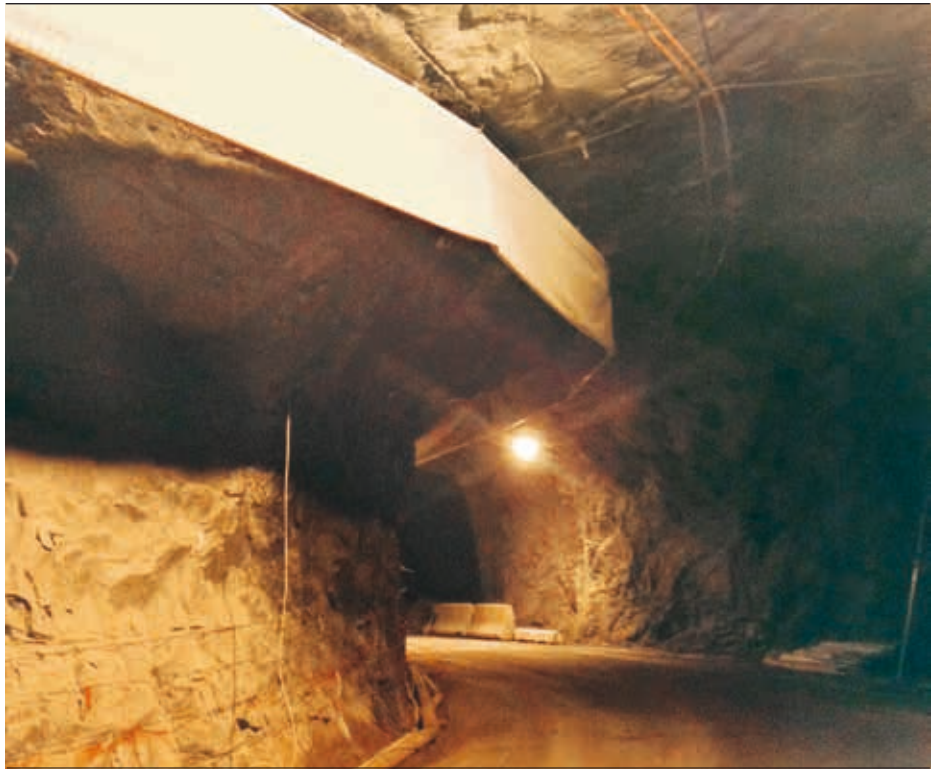
1 A ventilation duct in an underground mine
