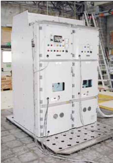
3 Seismic test arrangement on UniGear ZS1 during Doel NPP qualification
