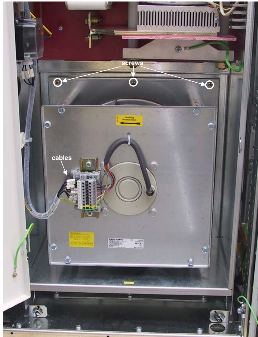
Figure 10-1 Converter fan in frame A6
