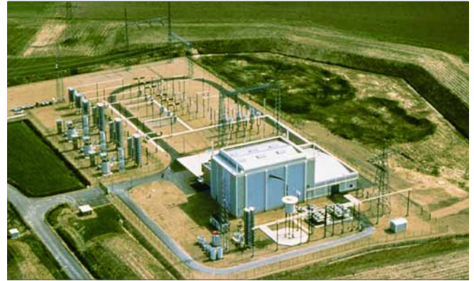
Baltic Cable HVDC converter station
