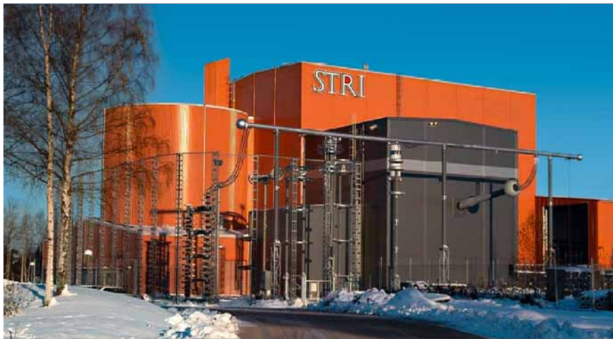
STRI laboratory in Ludvika, Sweden with 800 kV UHVDC test installation
