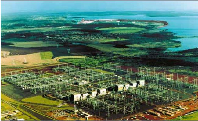
Foz do Iguaçu converter station with the Itaipu 12,600MW power station in the background
