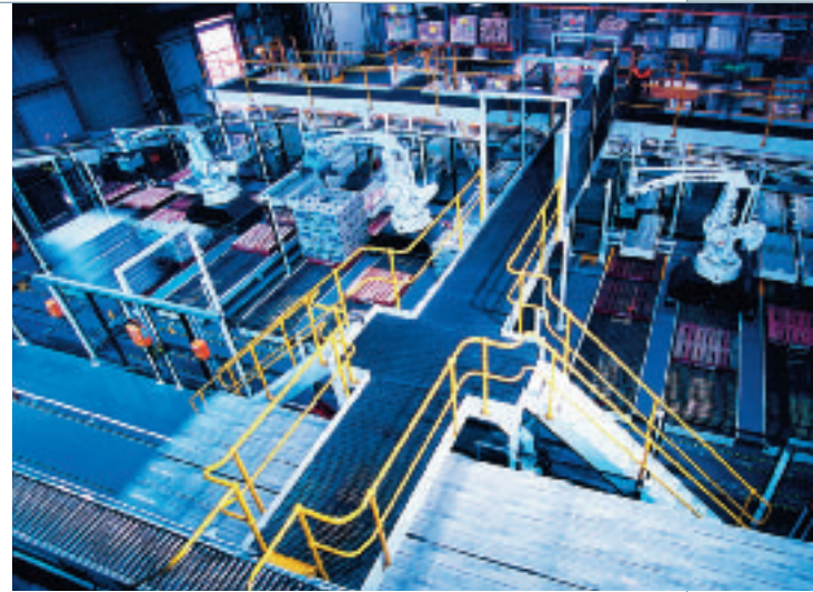
The robot-based palletizing solution at Arnott's Snackfoods' Sydney plant comprises four robots handling 12 product lines simultaneously.
