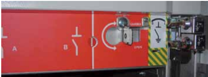
Figure 65: Front panel with operating slots of busbar-disconnector
