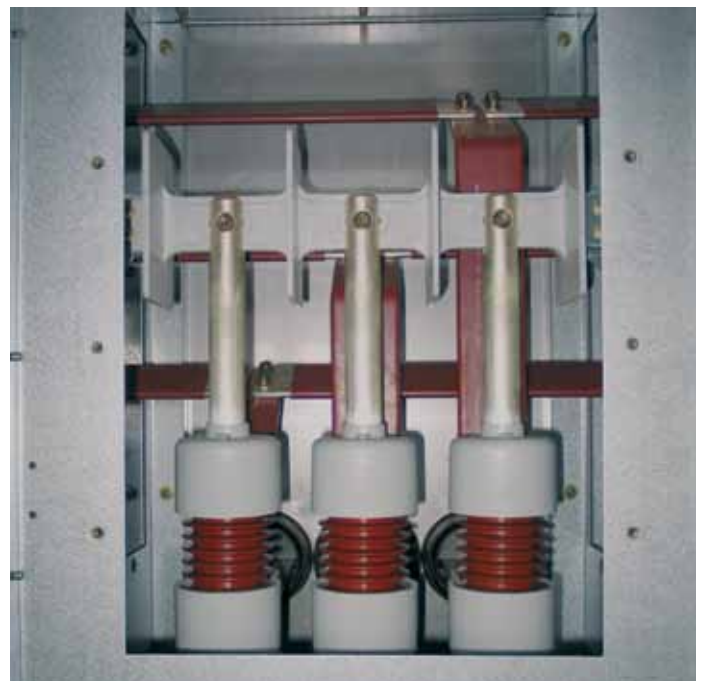
Figure 64: Open position of busbar-disconnector
