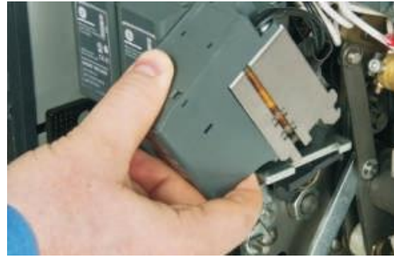
Figure 3. Coil Assembly
