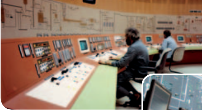
Figure 2: the old plant mimic versus the new extended workplace of ABB and CCR layout (pictures below)
