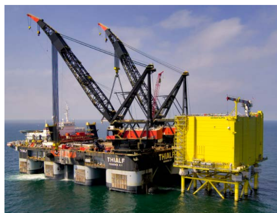
Figure 6 DolWin alpha installed
