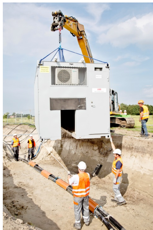
Figure 12 Jointing container
