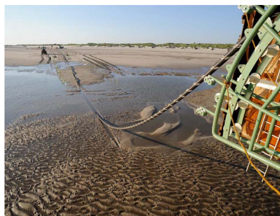
Figure 13 Cable pulling Norderney
