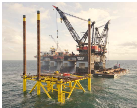
Figure 4 DolWin alpha jacket piling
