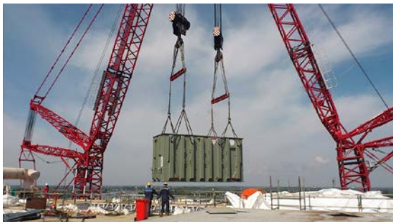
Figure 17 Lift of a power transformer onto DolWin alpha
