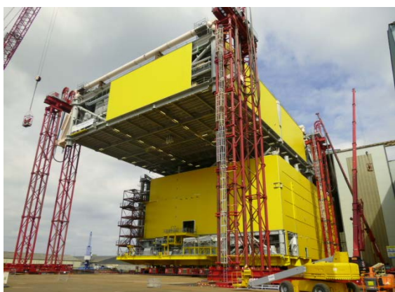
Figure 3 DolWin alpha "mating"
