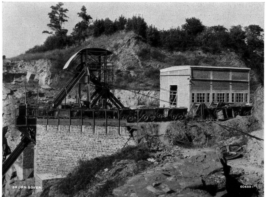
Fig. 3. — Upper terminal station of hoist and machine house with winch. The machine house contains the necessary equipment for automatic and manual control.
