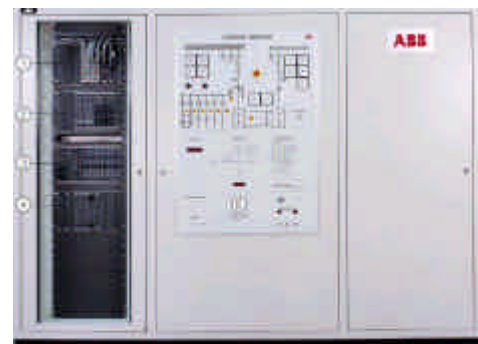
Cabinets containing the control system for the Bremen static frequency link
