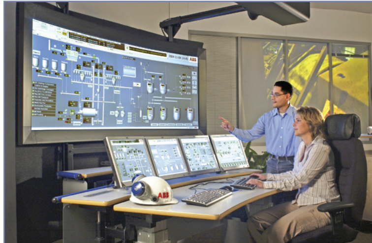
ABB's 800xa automation system can cover an entire mining operation
