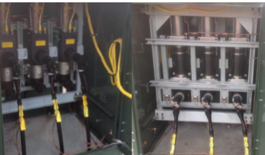
Elastimold MVI interrupters provided a dead-front and shielded solution that does not rely on oil, gas or air for insulation or interruption, resulting in long-life, maintenance-free\* operation.
