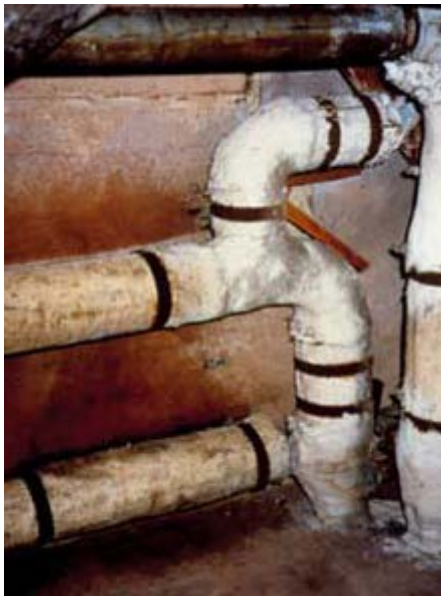
Photos 7&8 Damaged Asbestos Insulation on Pipe work (Source UK Health & Safety Executive "Asbestos Essentials")
