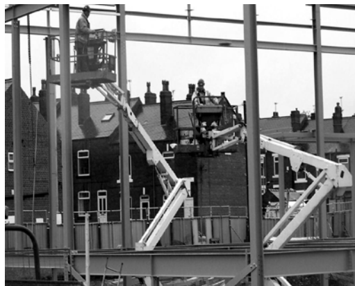
Fig 9 Potential for Collision if more than One MEWP is in use
