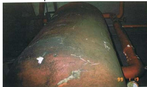
Photos of Damaged Asbestos Thermal Insulation
