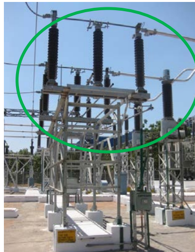
Fig 15 Isolator with Earth Switch
