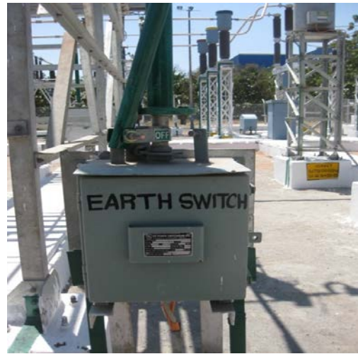
Fig 17 Earth Switch
