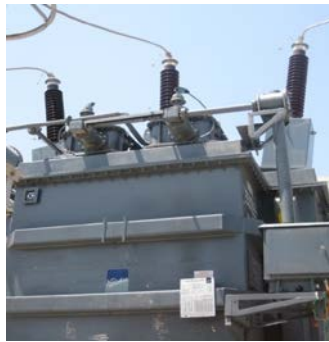
Fig 24 Power Transformer
