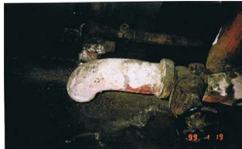
Photos of Damaged Asbestos Thermal Insulation
