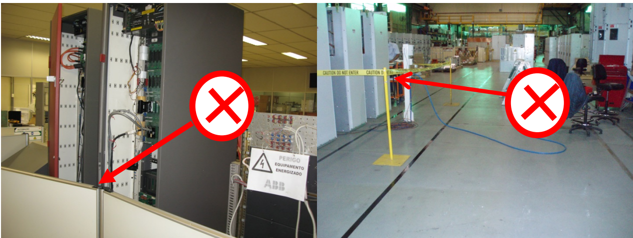
Figs 5 & 6 Improper Temporary Barriers
