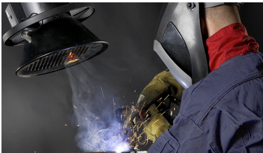
Fig 6 Example of Effective Local Exhaust Ventilation
