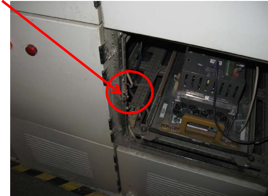
Fig 2 Production test Facility
