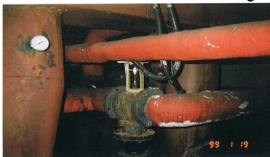
Photos of Damaged Asbestos Thermal Insulation
