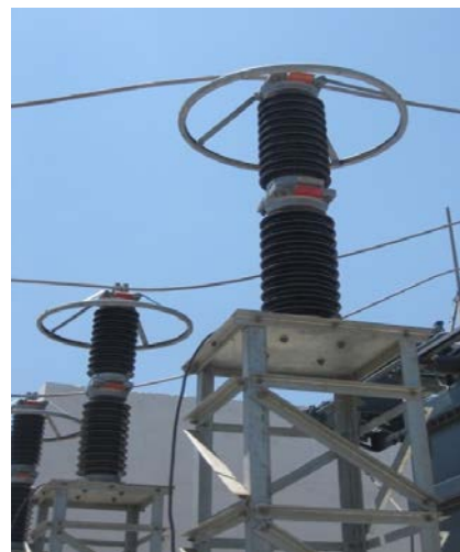
Fig 23 Lightning Arrester with Corona Rings
