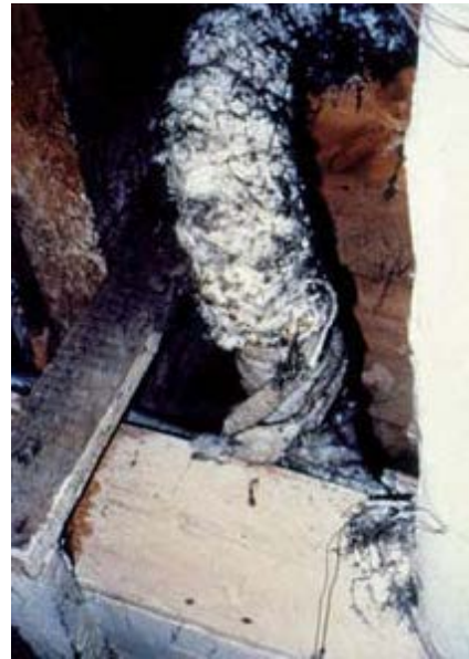
Photos 7&8 Damaged Asbestos Insulation on Pipe work (Source UK Health & Safety Executive "Asbestos Essentials")
