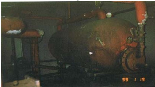
Photos of Damaged Asbestos Thermal Insulation
