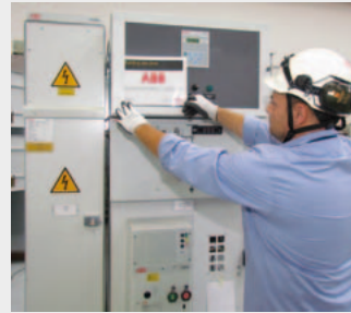
1. Clearly identify the work location
