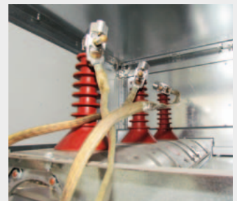
6. Carry out earthing and short circuiting
