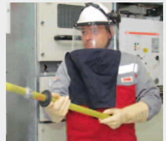
4. Take special precautions when close to bare conductors
