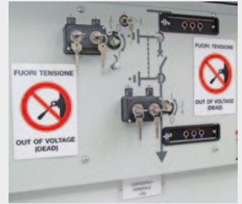
2. Disconnect and secure against reconnection
