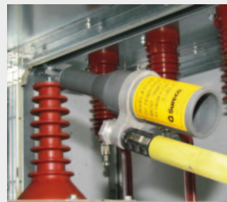
5. Check the installation is dead
