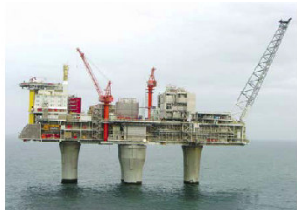
Troll A Platform with the HVDC Unit (Central)
