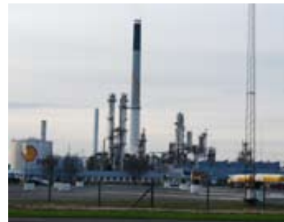
Shell's refinery in Fredericia (above) supplies a reasonably constant quantity of excess heat, as do the waste burning plants in Kolding and Middelfart. Fluctuations in the load are dealt with by supplementing the heat from the Skærbæk plant with local peak and reserve production.
