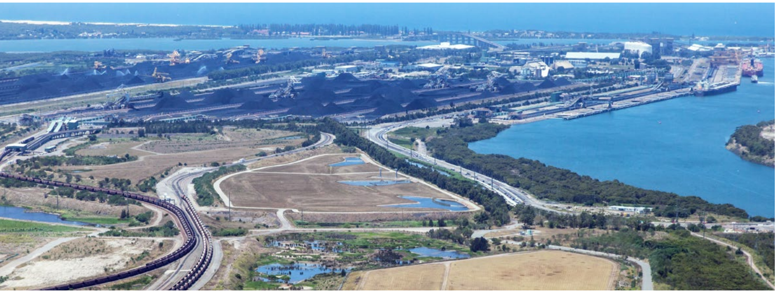
— Coal export terminal on Kooragang Island, New South Wales, Australia.
