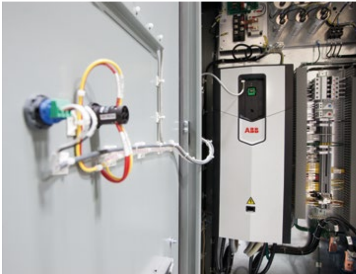
The ACS880 variable frequency drive solved the MagnoDrive performance problems at low rpms.
