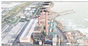
ABB has designed and commissioned CHP projects around the world. One is at the heart of a district heating system in China that takes heat normally wasted in a cooling tower and uses it to heat homes for about one million people, reducing  $CO_2$  emissions by 500,000 metric tons and  $SO_2$  emissions by 2,200 metric tons annually.
