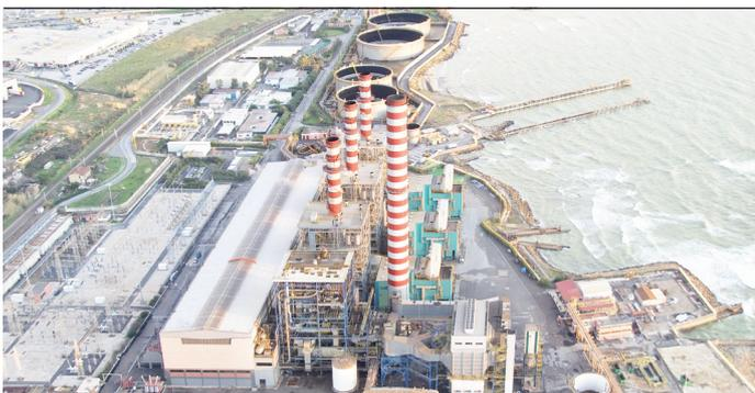
ABB has designed and commissioned CHP projects around the world. One is at the heart of a district heating system in China that takes heat normally wasted in a cooling tower and uses it to heat homes for about one million people, reducing CO<sub>2</sub> emissions by 500,000 metric tons and SO<sub>2</sub> emissions by 2,200 metric tons annually.
