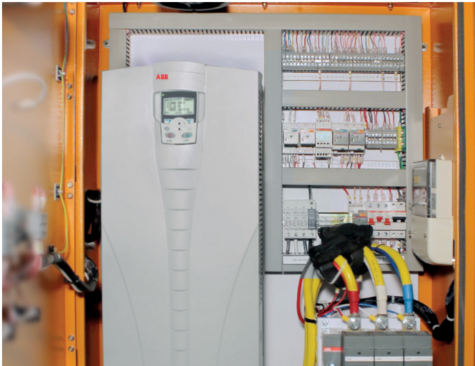
The drives were installed close to the pump's motors and configured to automatically restart when needed. This reduced the manpower required to operate the irrigation system.
