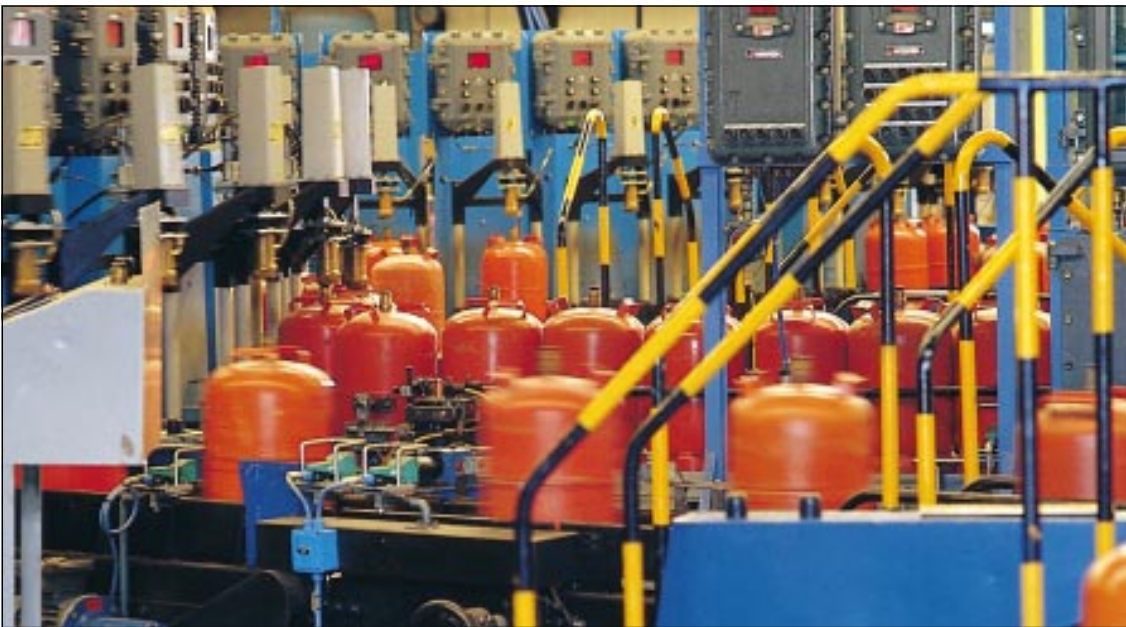
One of the two carousels at a bottling bay in the Pinto distribution centre. Filling of a gas bottle takes 1.5 or 2.5 seconds depending on the type.
