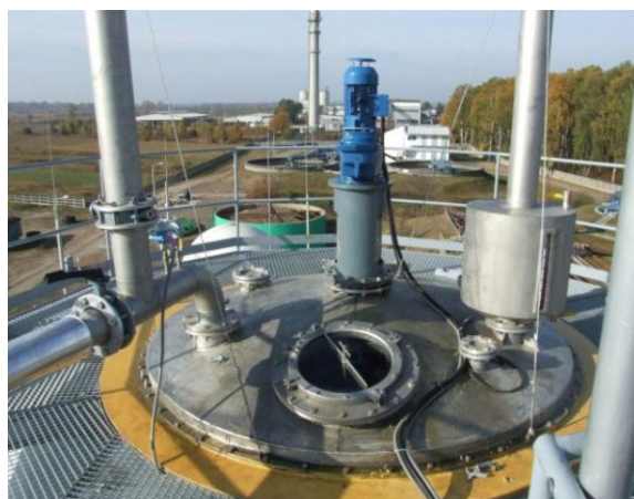
01 Control of foam level in a fermentation chamber
