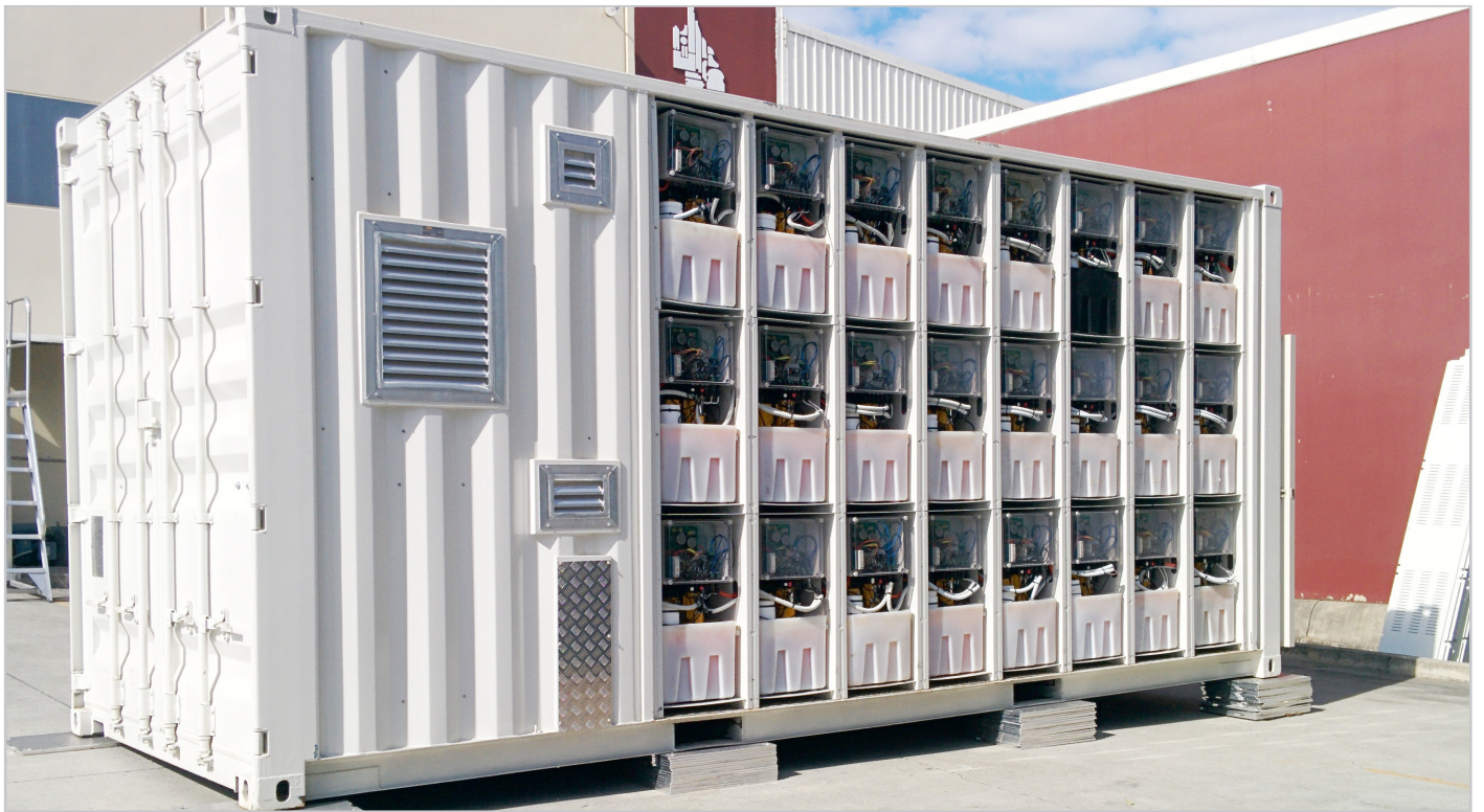
PCS100 ESS successfully applied with a zinc bromide flow battery at Redflow in Australia
