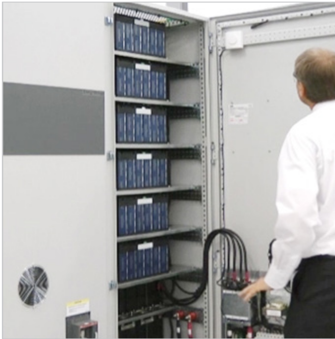
LS Mtron ultra capacitor module installed in PCS100 UPS-I Industrial UPSs
