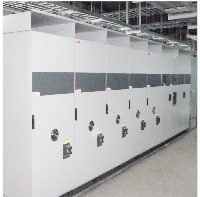
A PCS100 UPS-I installation with ultra capacitor storage in a semiconductor facility
